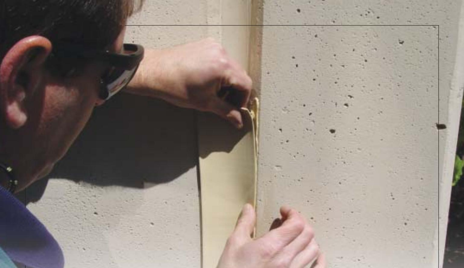
A close-up photograph of a construction worker wearing safety glasses and a blue shirt. The worker is using a caulking gun to apply a thick, yellowish sealant into a vertical joint in a light-colored concrete wall. The worker's hands are visible, one holding the caulking gun and the other supporting the wall. The background is a plain, textured concrete surface.
