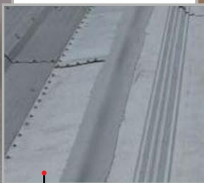
Figure 2: Precured silicone sealant used to seal between a new addition and an existing metal building
