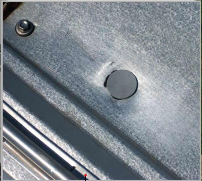
Figure 6: A hole in a roof deck repaired using precured silicone sealant
