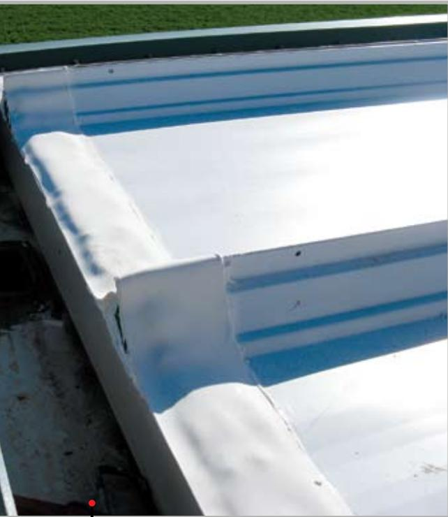
• **Figure 7: The repair of a metal roof using precured silicone sealant**
