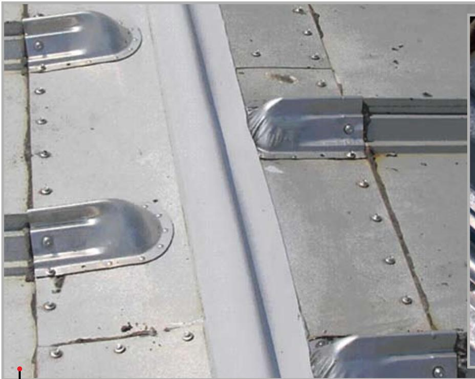
Figure 5: Precured silicone sealant used in a ridge repair application
