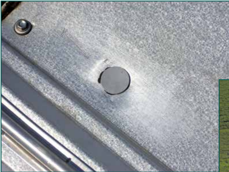
Figure 9 – Hole in a metal roof deck repaired using precured silicone sealant.
