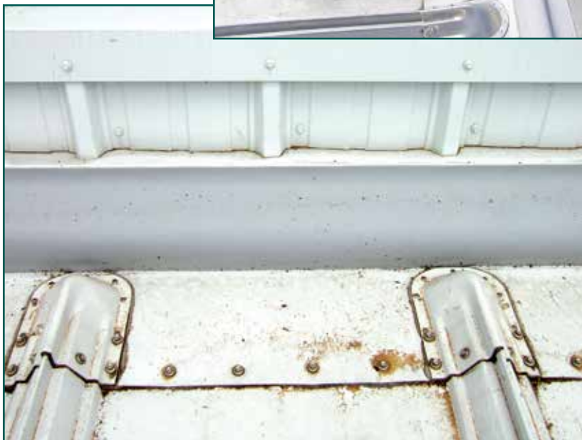
Figure 8 – Precured silicone sealant installed in a metal roof-to-wall transition application.
