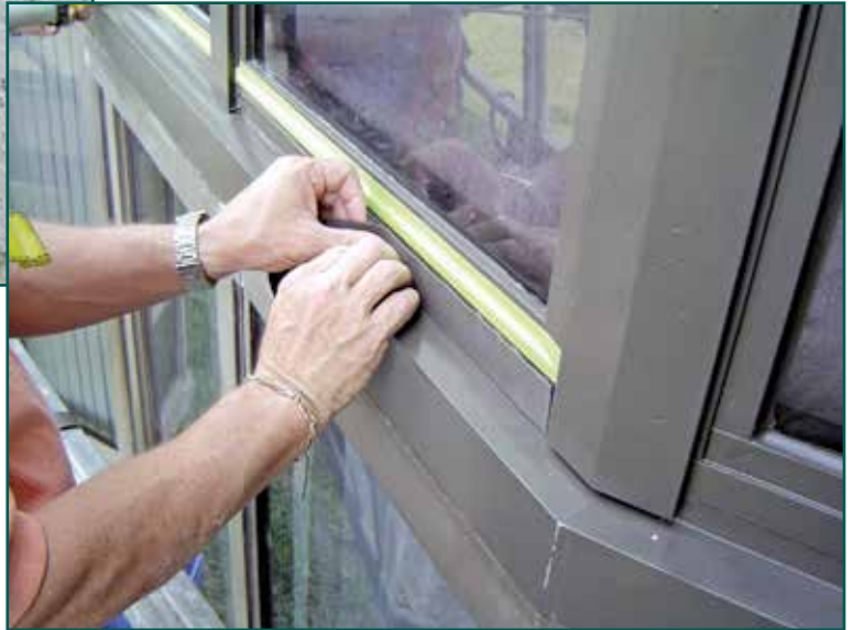
Figure 5 – Pre-cured silicone sealant installed in an aluminum window system.
