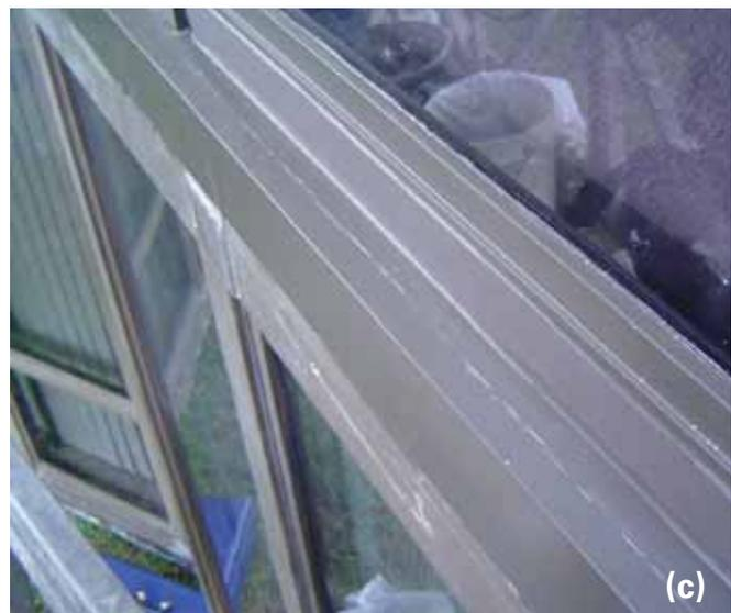
One of the biggest advantages of using pre-cured sealants in these applications is that, because they can be installed directly over the existing failed sealant and the old sealant does not need to be removed, labor cost savings can be significant. Several of the most common building envelope repair applications include:
