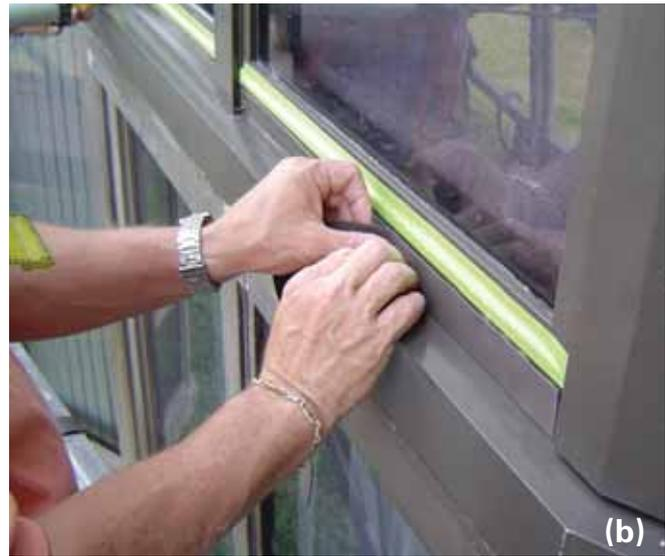
The basic steps involved in installing pre-cured sealant include the application of the adhesive (a), pressing the pre-cured sealant into place (b) and the completed installation (c).
