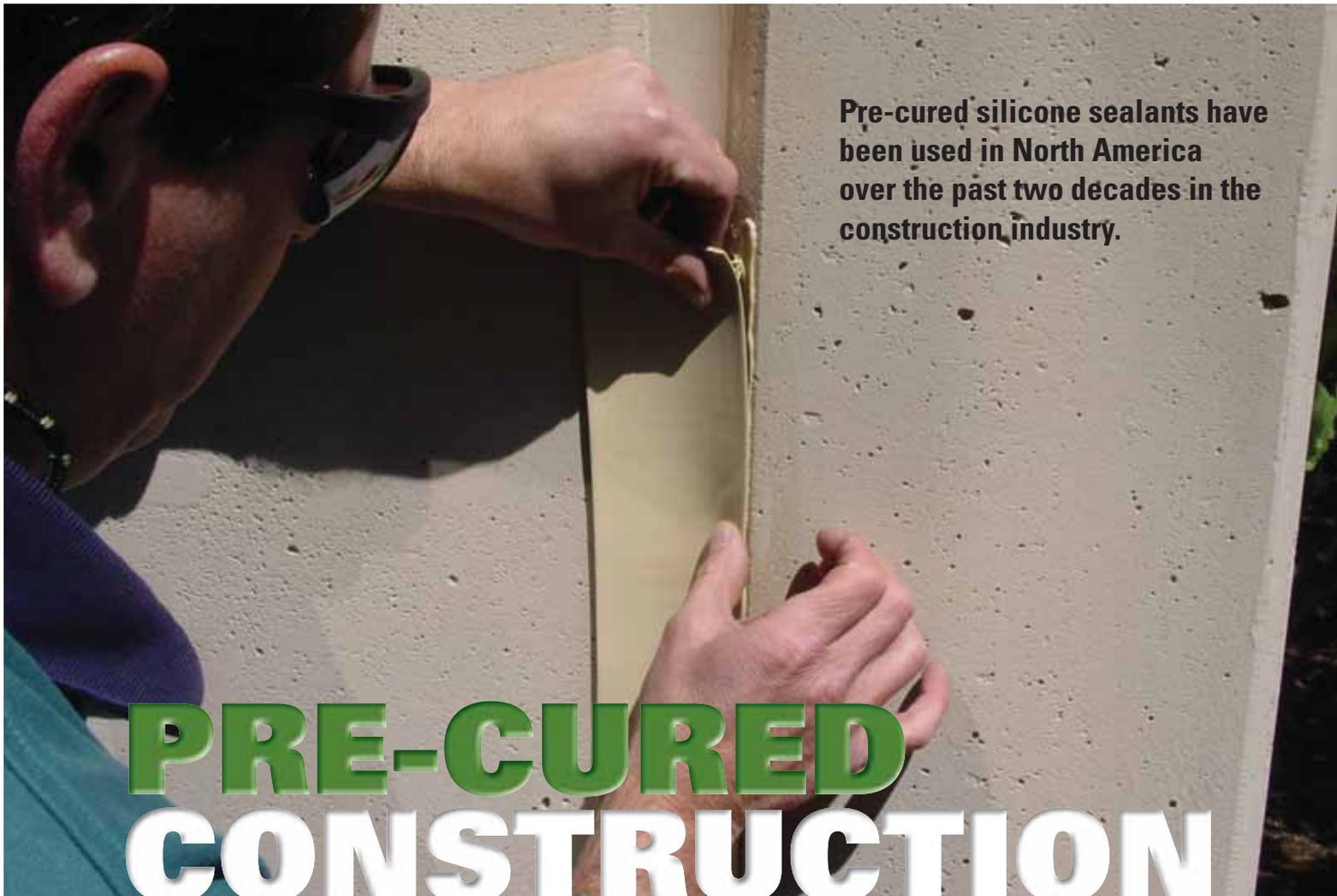
**Pre-cured silicone sealants have been used in North America over the past two decades in the construction industry.**
