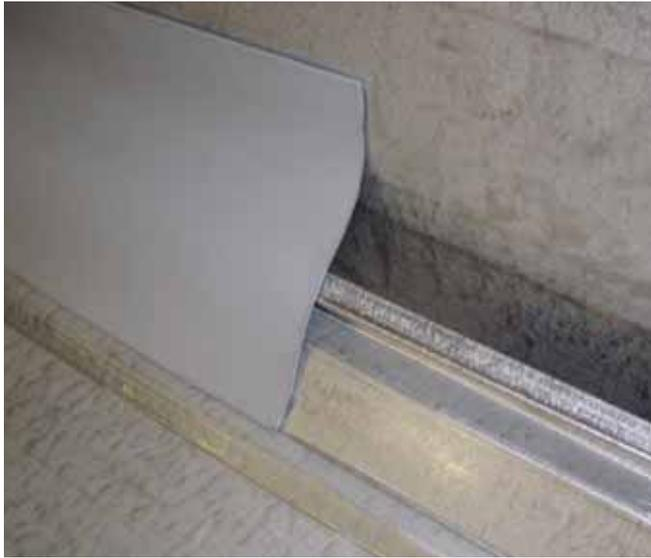
One of the most important features of pre-cured sealants for metal building applications is the fact that no mechanical fasteners are required for installation.
