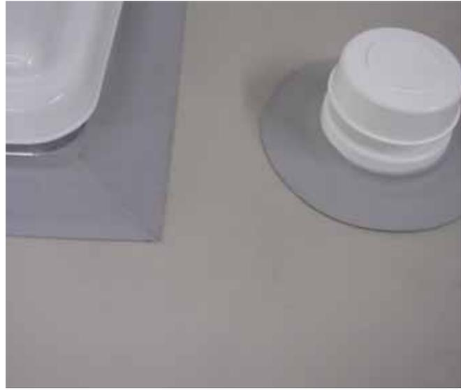
Pre-cured sealants can be easily cut to seal straight or rounded penetrations, including vents, windows and doors.
