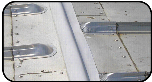
ImmerSeal® in a ridge in a repair application
