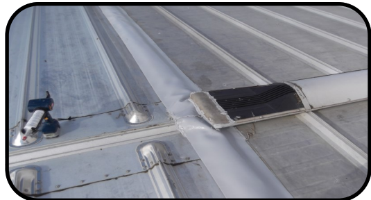
ImmerSeal® HD used to seal a roof joint between a new and existing building
